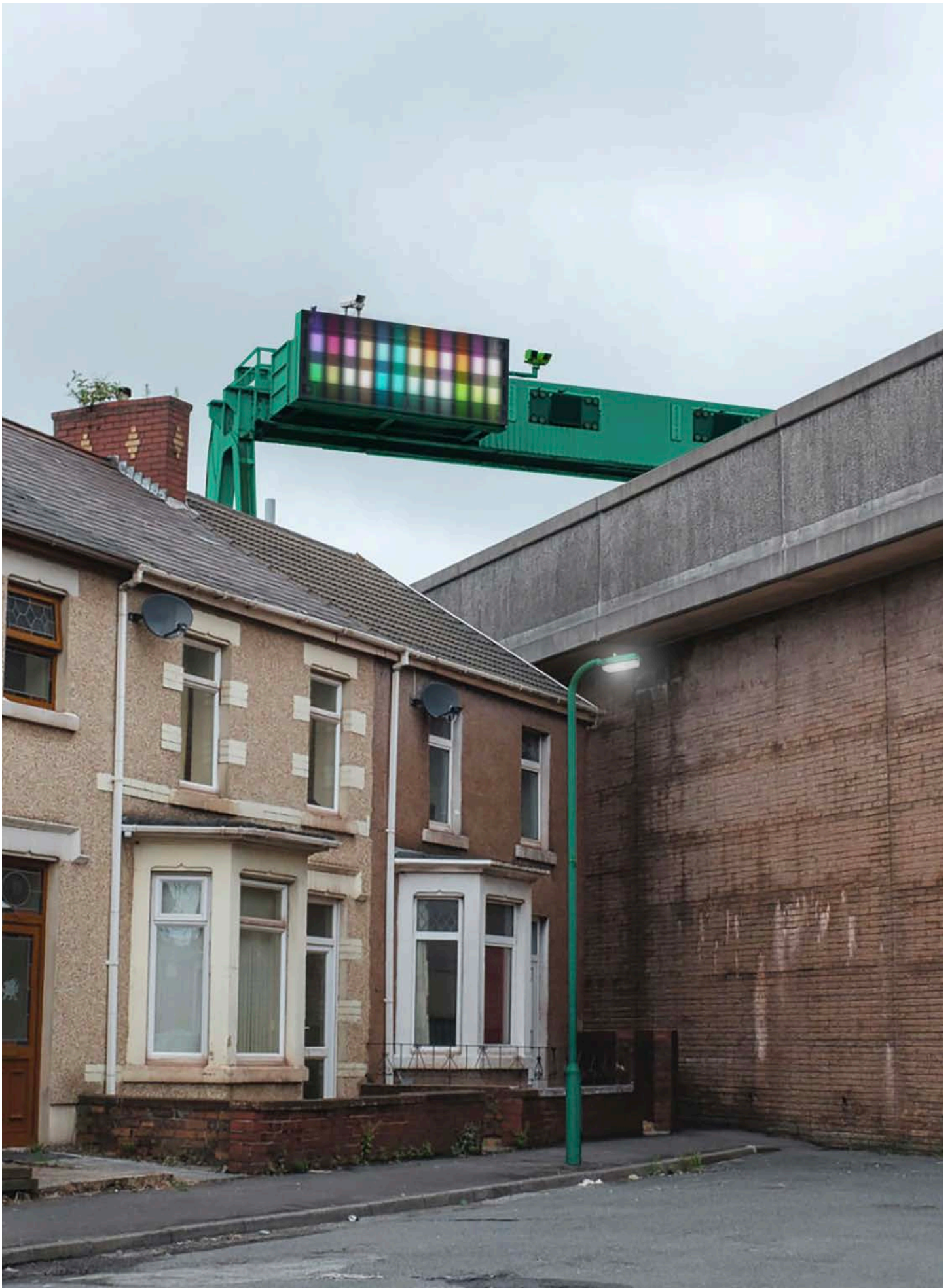
vii M1 through Port Talbot / highlighting the identity changes to the infrastructure that makes up Port Talbot
